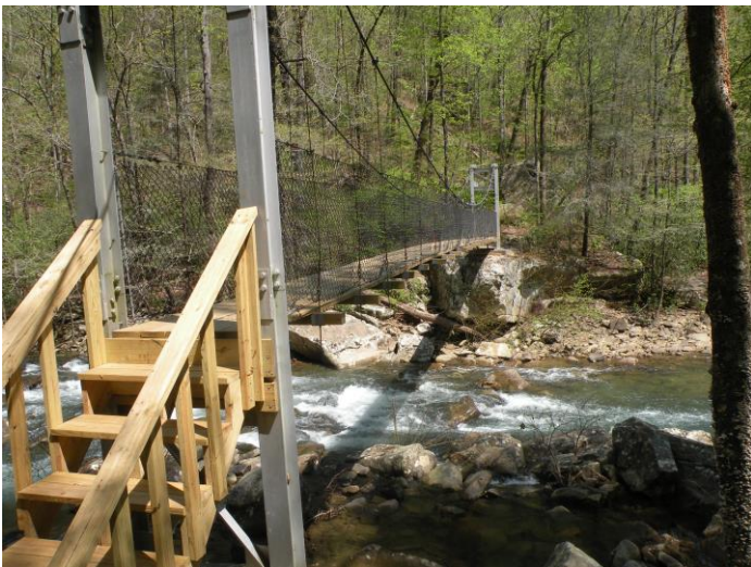
Big Soddy Bridge on Cumberland Trail (TN)
