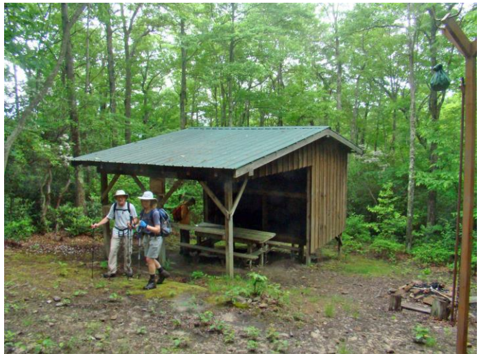
Adena Spring Shelter on Pine Mountain Trail
