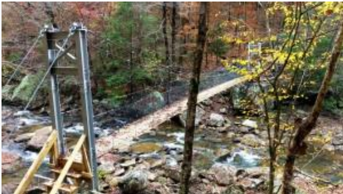
Big Soddy Bridge Opens November 2015 (photo Shauna Anschuetz)
